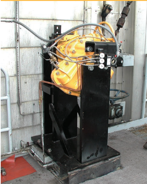
ID bypass drive that produces 5,000 ft-lbs of torque
